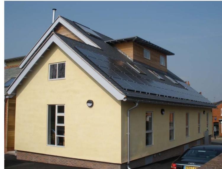
Image 2 – Photovoltaic and solar thermal array
