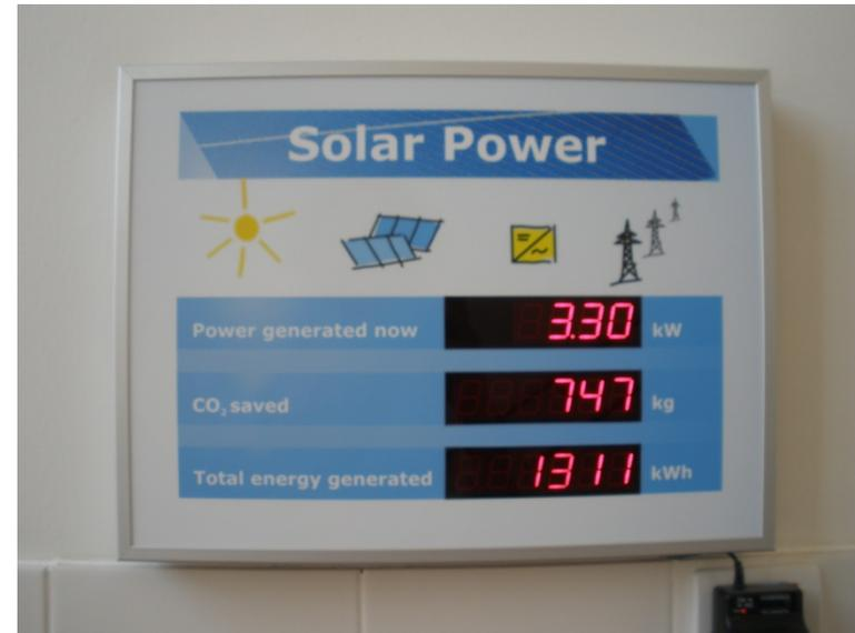
Image 4 – Real-time display of photovoltaic output
